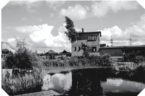
In the summer of 2022, the artists also lived on the first floor of the administrative building, which had been empty for several decades.
